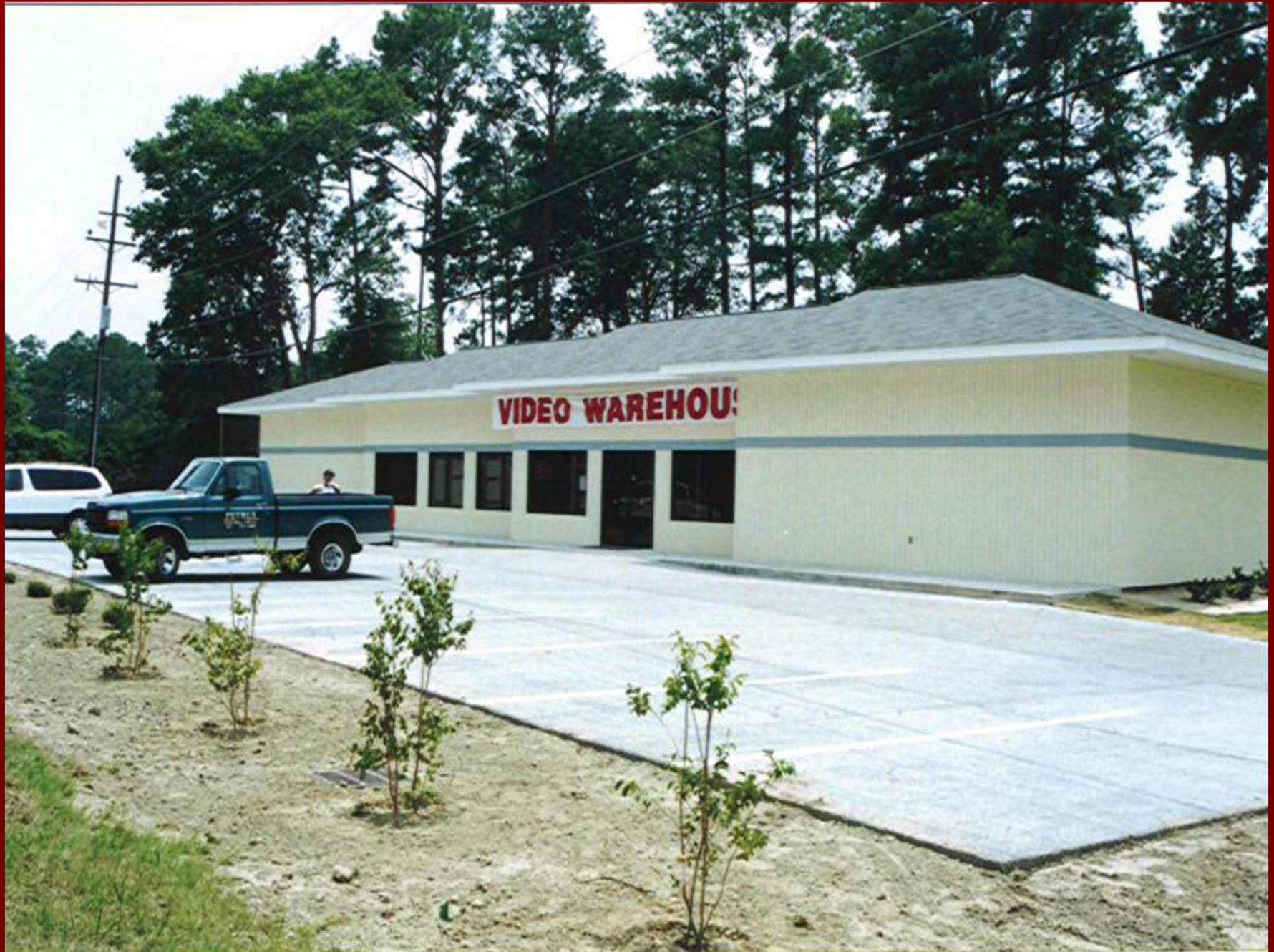
Video Warehouse - Rincon, Georgia - Pervious Paving Stormwater Management
